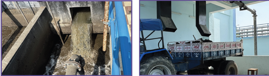
Figure 17: Inlet WW Chamber from Households and Transportation of Sludge
